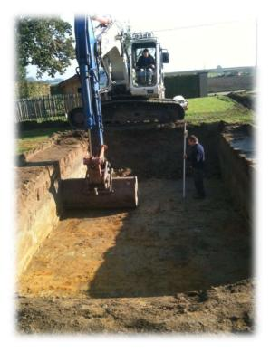
Important: If there is a risk of ground water, provision must be made in the base to drain/pump it away from the pool.
