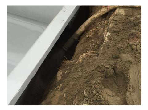
The pool can now be backfilled in layers until the aggregate is level with the lower fibreglass lip of the pool which will form the base for the pool surround coping stones.
