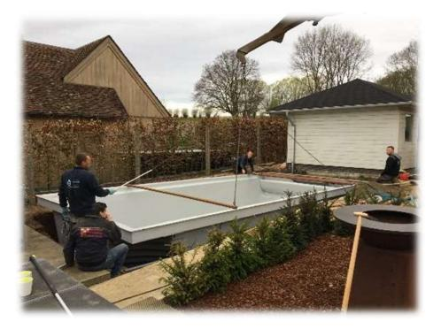
Ensure that the pool is level with use of a Laser Level.
