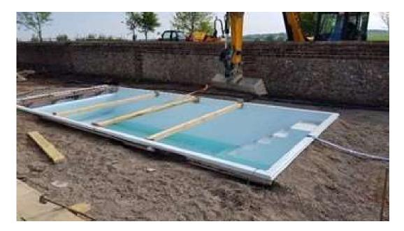
The braces can be removed ONLY after the pool water has reached operating level.
