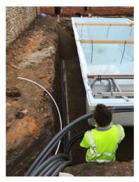
Notes: All pipework connections on the shell are 50mm pvc.
