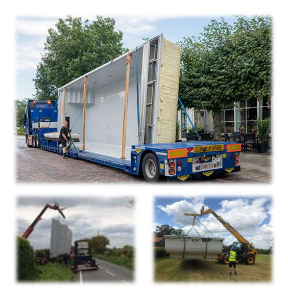
You will need to ensure that your chosen offloading vehicle has straps and/or chains that can be used for the lifting process. They are <u>not</u> provided with the delivery lorry. In the case of the pools delivered on their sides the pool is lifted from the lorry using the straps attached to the two reinforced lifting points. It is then moved to an area where the pool can be gently laid flat.
