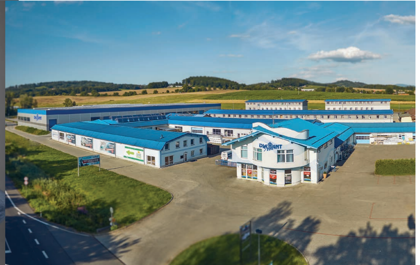
In 2020, a new 7,000 m 2 production hall for stainless steel pools was completed and all production is carried out at our 17,000 m 2 site in Valašské Meziříčí.
